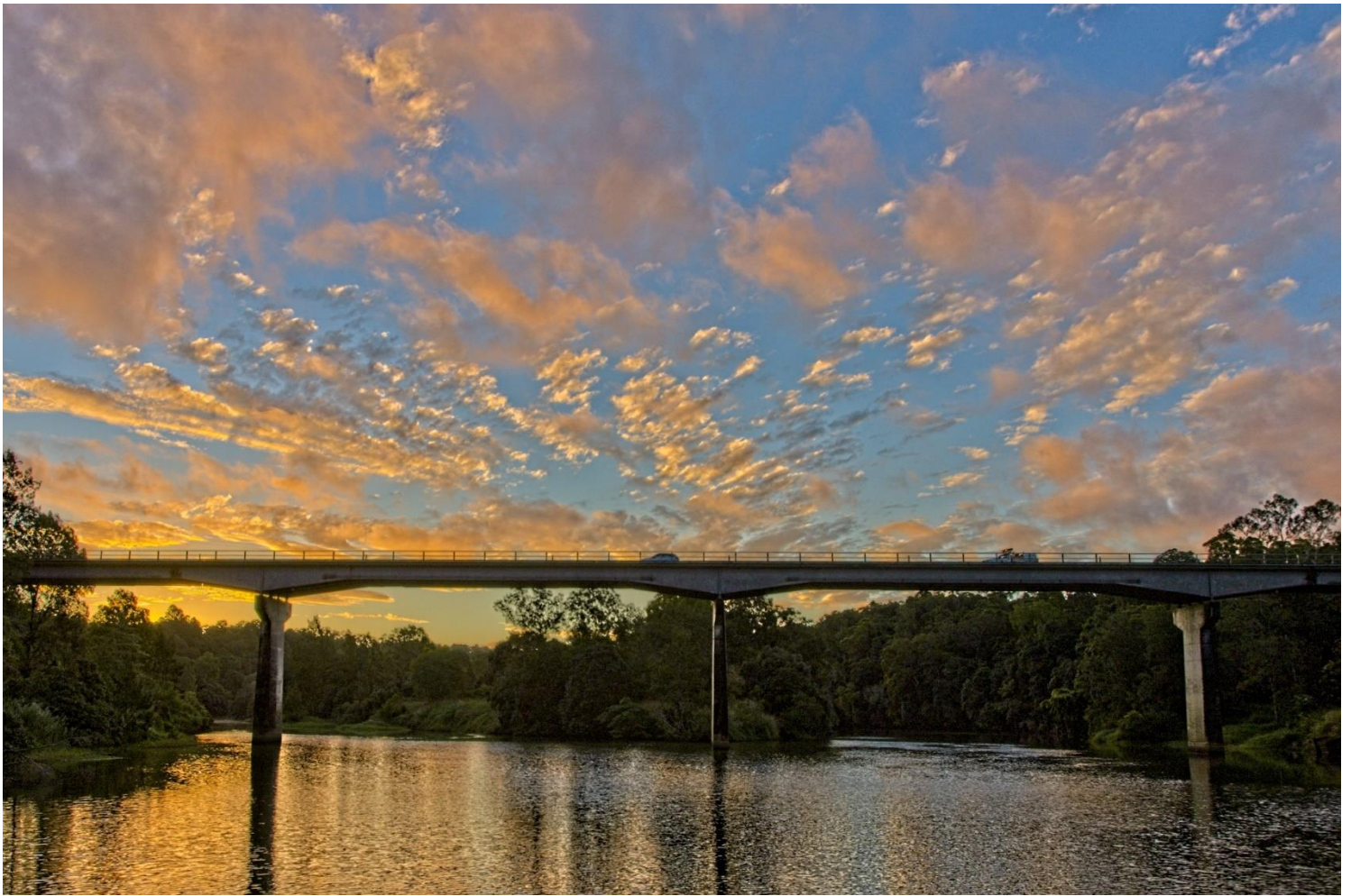
Image: Barron River bridge near Kuranda. © State of Queensland.
