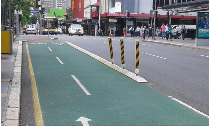
Figure 4.1.2(c) – Gympie Road at Kedron Park Road southbound, Kedron Park (plastic kerb with vertical delineators)
