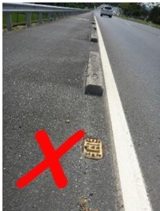
Figure 3 – Example of historical concrete barrier kerbs
