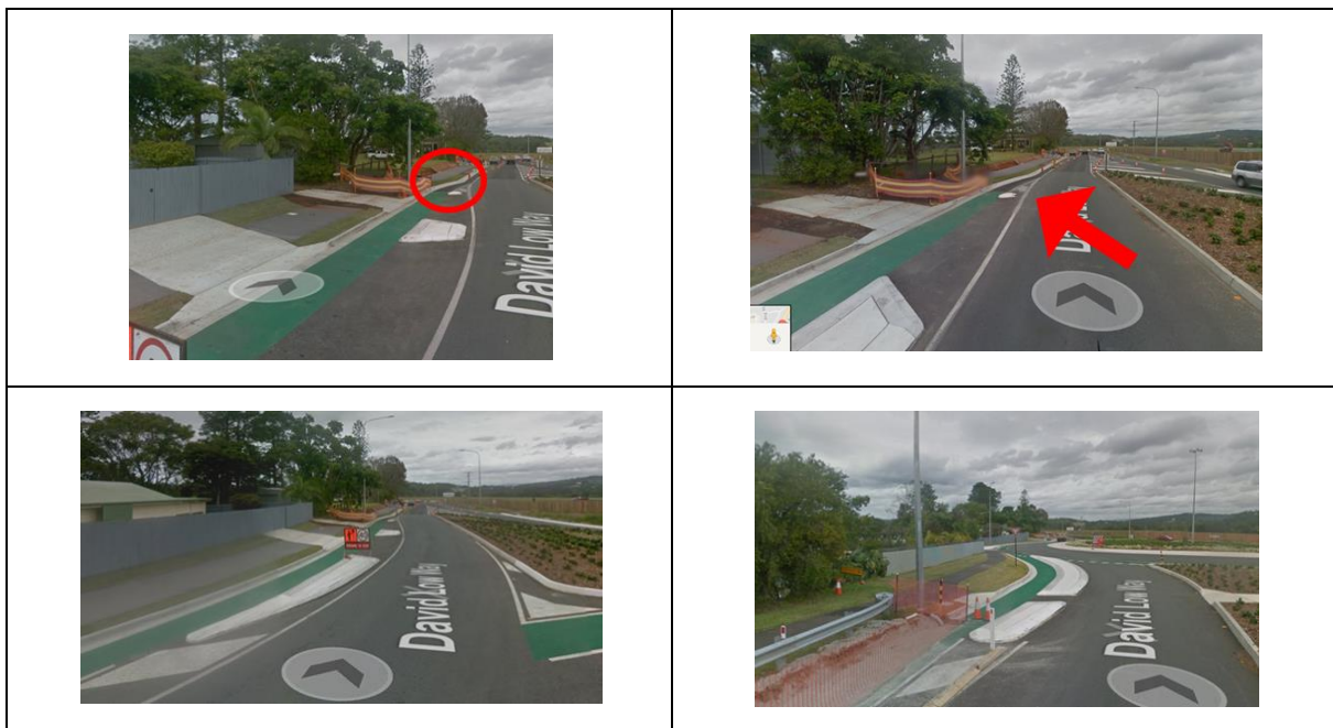
Figure 4.1.1 – David Low Way: Showing concrete islands separating the bicycle lane from the road
