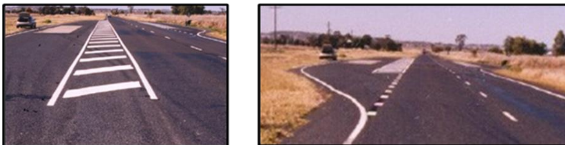
Figure C.2 – Line marking of operational separation area
