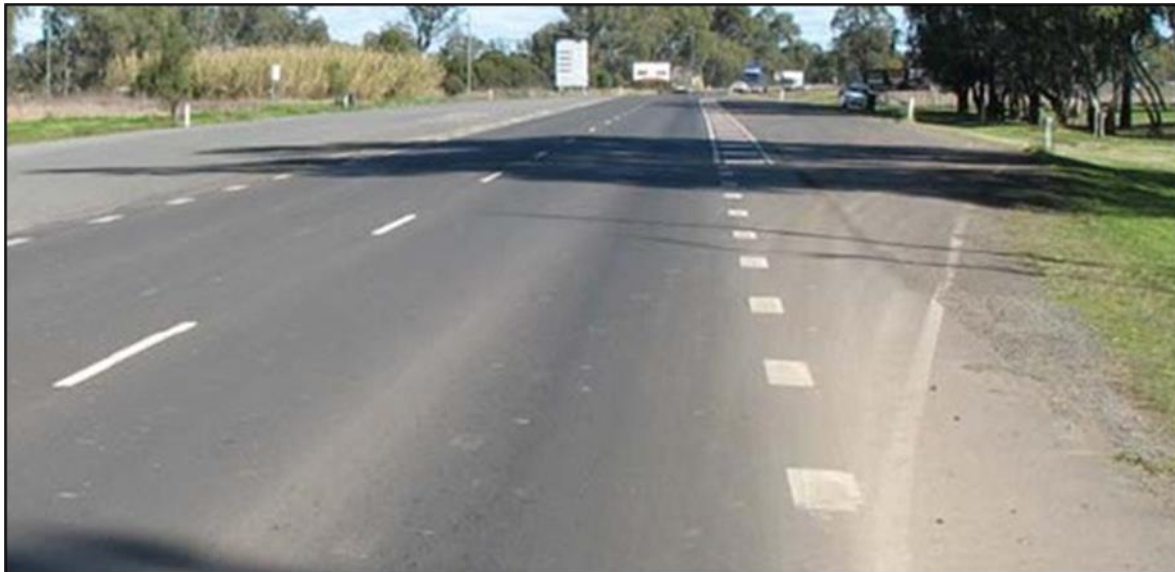
Figure 8.2.2 – Roadworks site edge definition line
