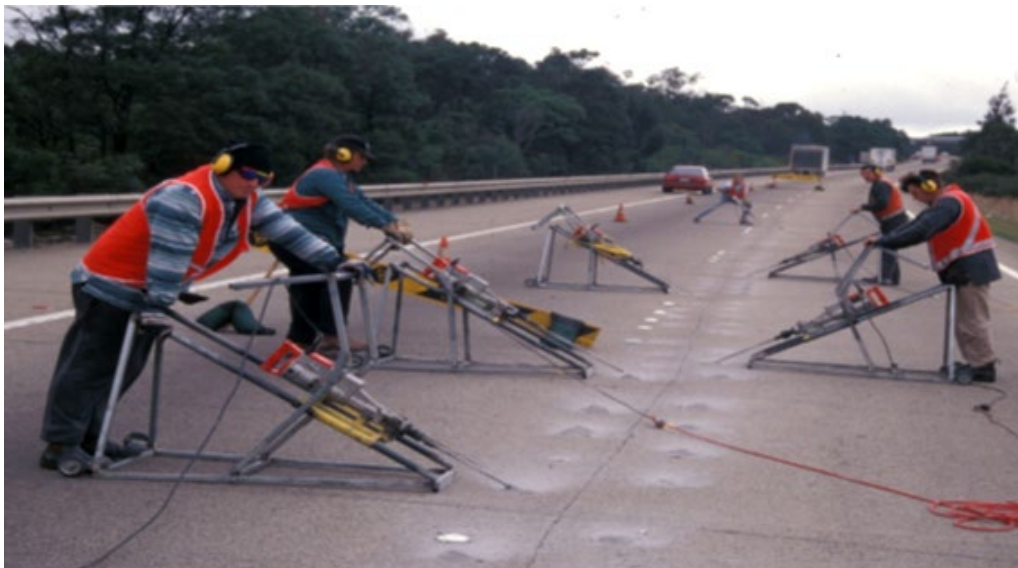
Figure 7(c) – Cross stitching of longitudinal crack
