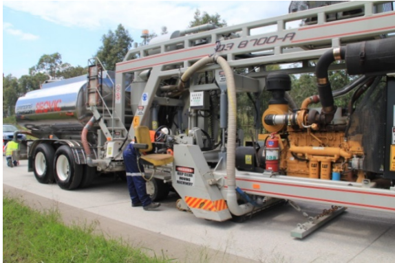
Figure 7(h) – Diamond grinding in progress
