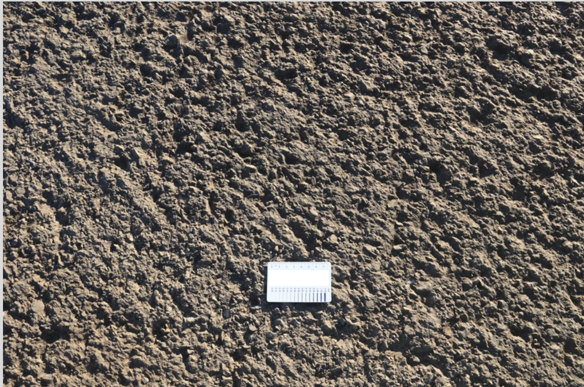
Figure 8.8.9.4.2(b) – Example of an acceptable hard-cut surface
