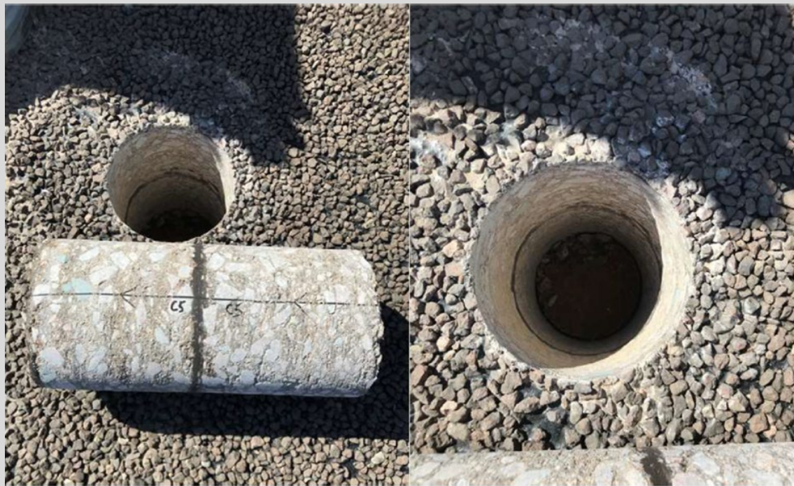
Figure 8.8.9.4.3 – Core showing the C170 spray seal interlayer bonding plant-mixed foamed bitumen stabilised layers together
