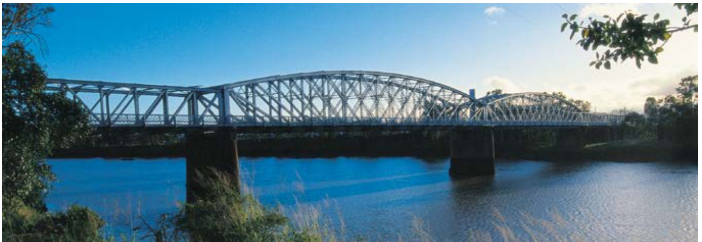
Alexandra Railway Bridge
