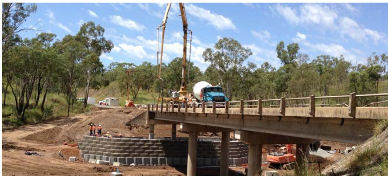
Reconstruction works on the Dawson Highway, Collards Creek
