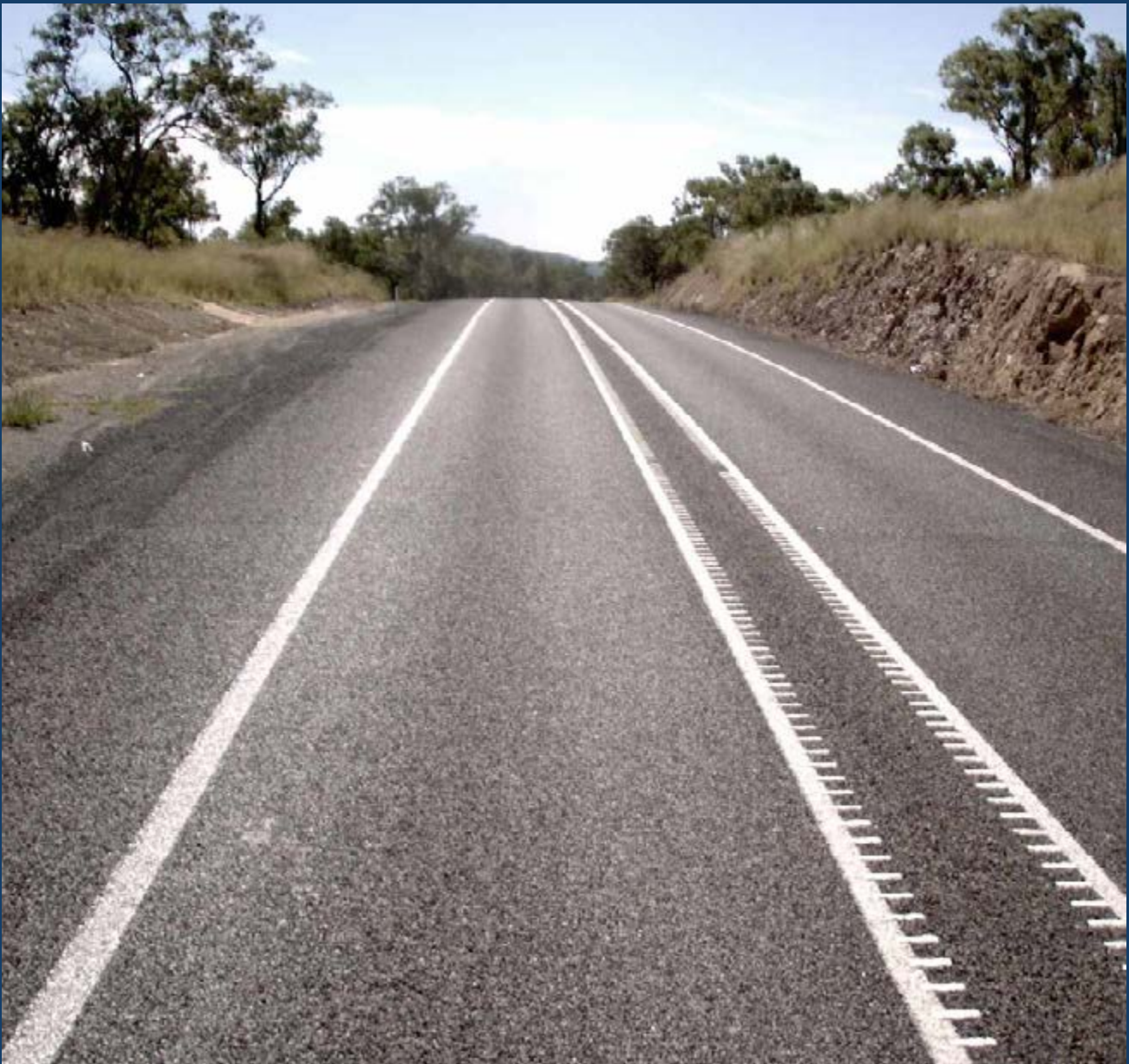
Wide centreline treatment, Bruce Highway, Gin Gin
