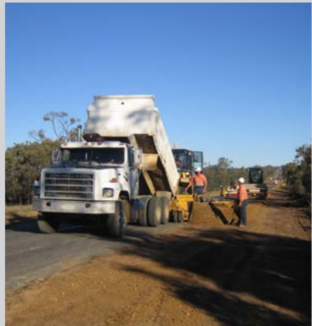
Road rehabilitation west of Calliope
