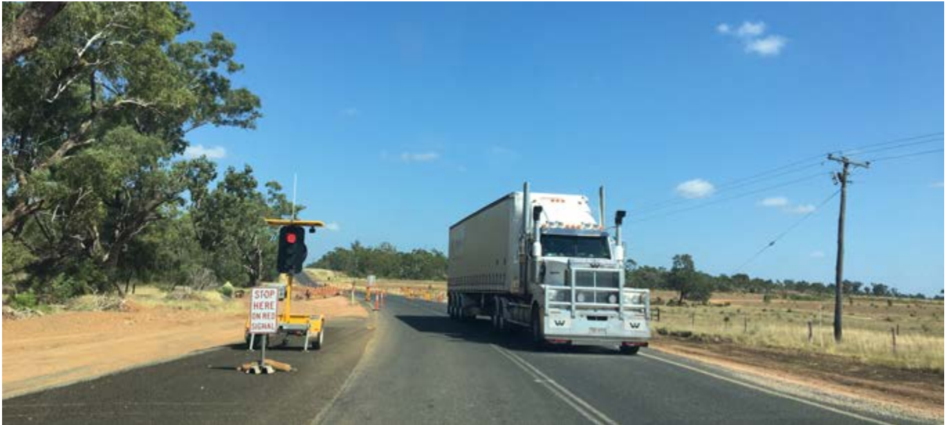
Heavy vehicle passing through road works
